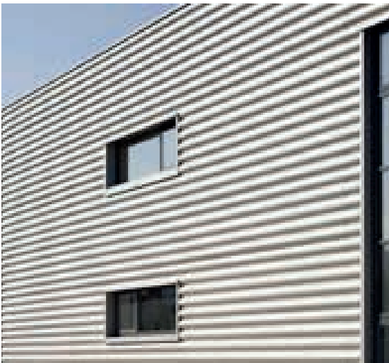
Metal Sheet Cladding
